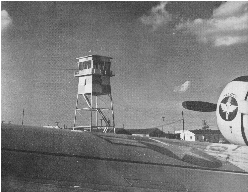
Malden AB control tower. (USAF photo)
